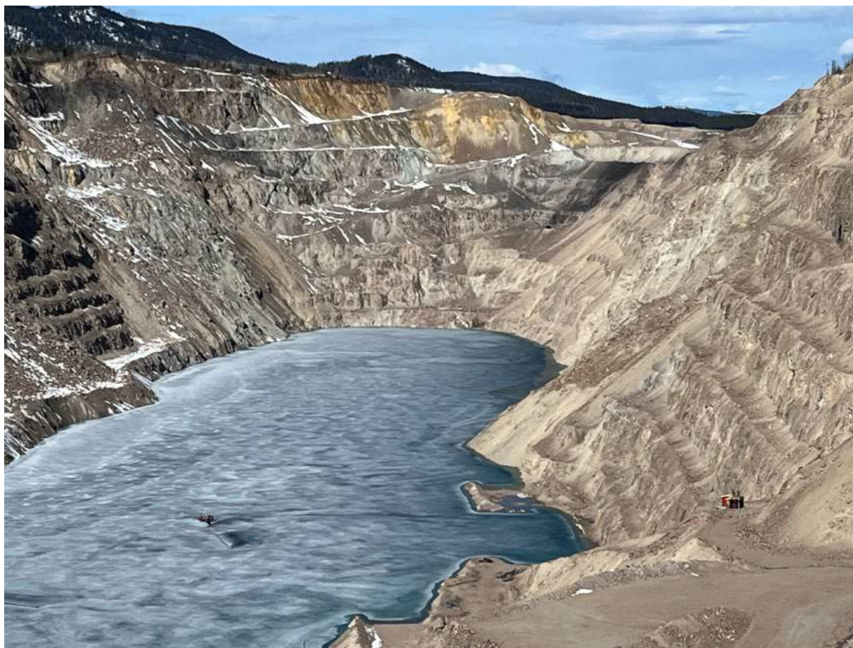
Figure 14.47 View of Endako Pit Showing Sloughing Source: AMPL, 2025
